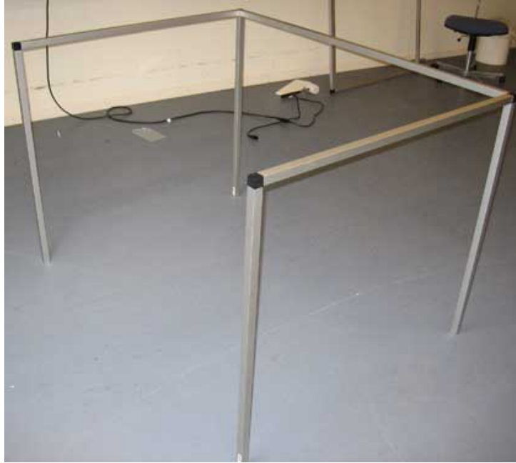
Step 3: Here the frame for supporting the glass screen frame is assembled.
